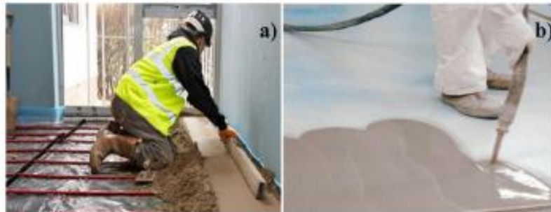
Figure 2.1. (a) Traditional semi-dry cementitious screed (b) Self-leveling mortar [1]
