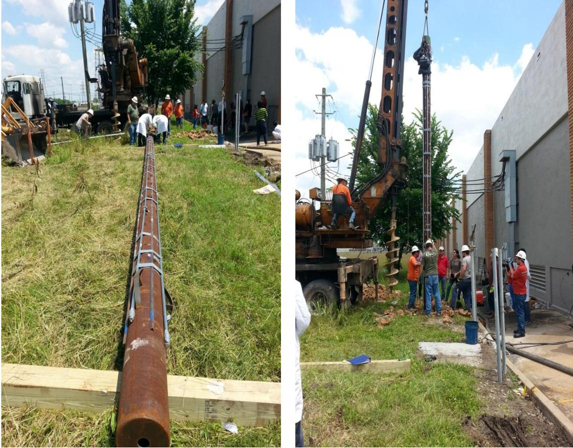
**Figure 3-14: Actual casing with wire combination before placing in the wellbore**
