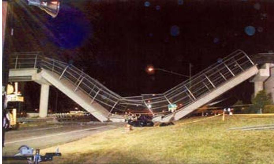
Figure 2.4 Collapsed pedestrian bridge
