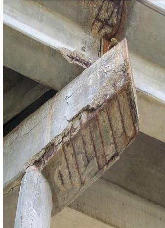
(a) Concrete cracking and spalling in bridge (TxDOT)
