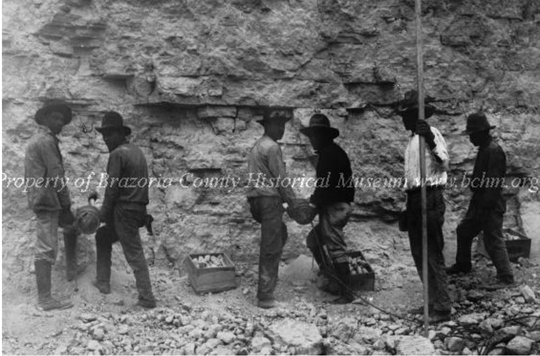
Seven-man crew setting dynamite charges in a giant block of extracted sulfur at Bryan Mound, Brazoria County (With permission of Brazoria County Historical Museum, 2022.024p.002, Nat Hickey Collection).
