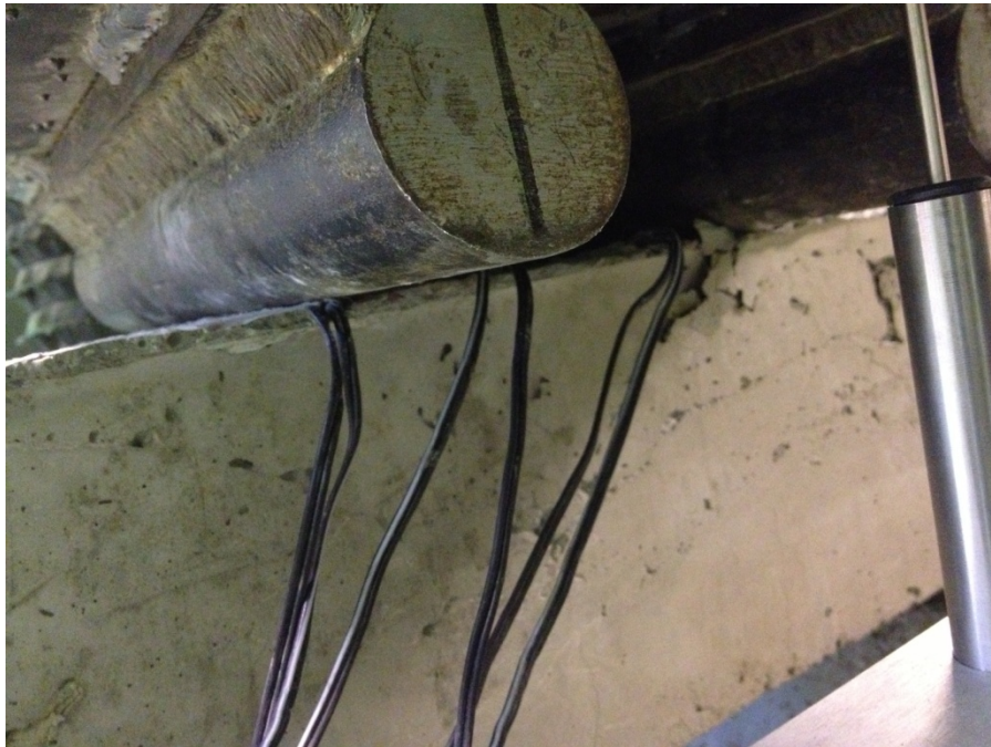
Fig. 7.14 Crack at Loading Point with Loading Equipment in Place
