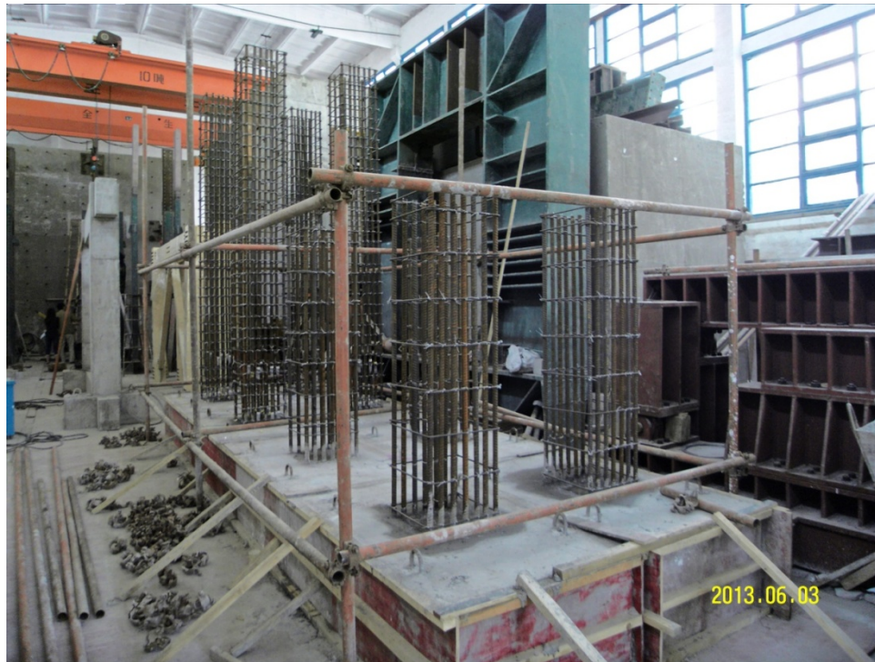
Fig. 8.4 Column Rebar Cages and Foundations
