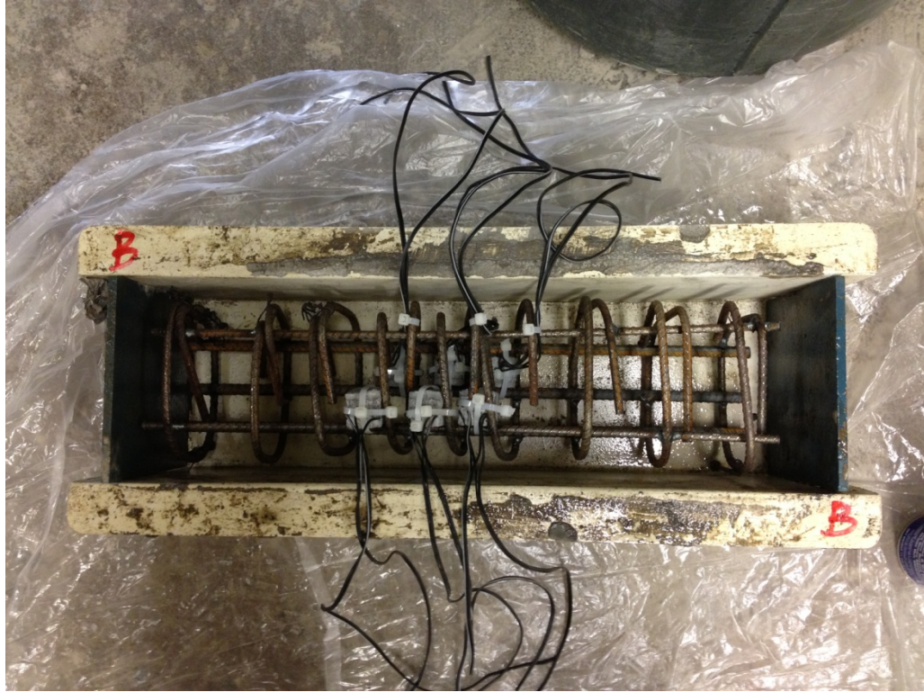
Fig. 7.4 Installed CNFAs and Beam Rebar Cage in Formwork
