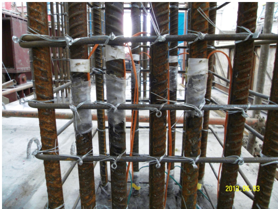
Fig. 8.6 Installed Thermocouples (Blue) and Strain Gauges (Orange)
