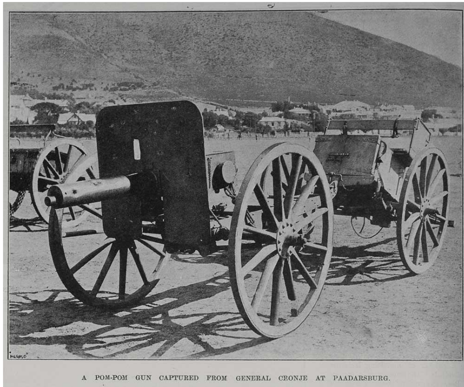
Figure 40: A Vickers-Maxim “pom-pom” gun, nicknamed for the sound it made when fired. 269
